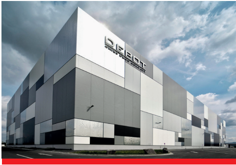
Foto: Gries Deco Company
